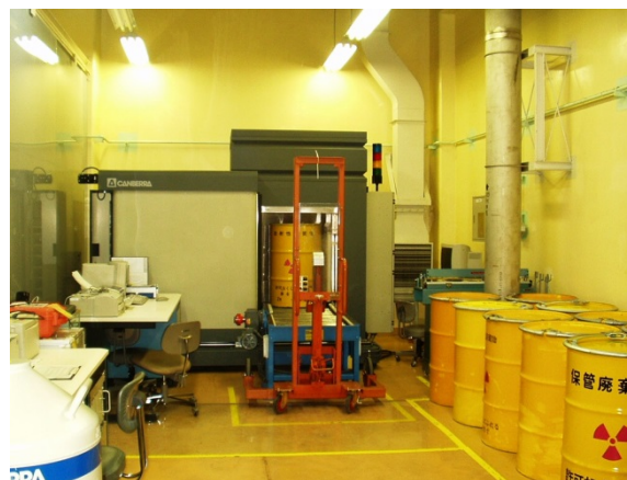
Measurement system of waste drum
